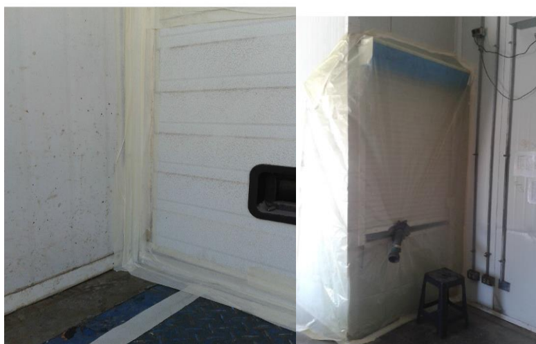
Picture 4. Sealing of doors using PVC tape and polyethylene sheeting.
