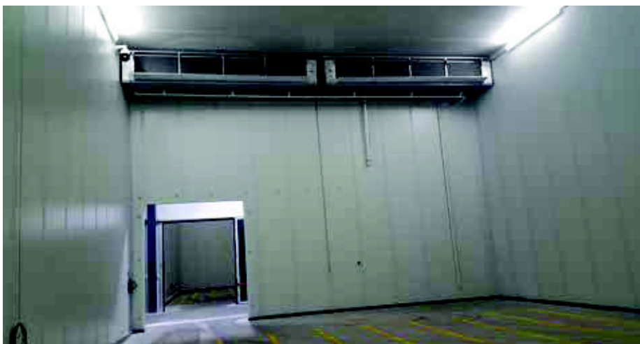
Figure 1. Due to treatment durations that are long, relative to those for methyl bromide, cold-storage phosphine fumigations can be conducted in large controlled-atmosphere rooms, maintained under cold-storage conditions, as a means to minimize disruptions to export throughput.
